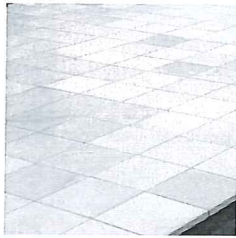
2. Natural stone paving within public square
